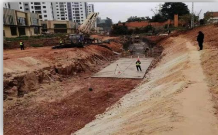
排洪沟沟槽开挖、边坡石方清收
